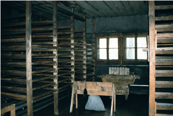
Figure 33. Drying room with drying tray racks.
