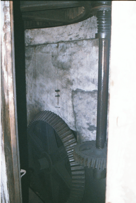
Figure 17. Water wheel gear.
