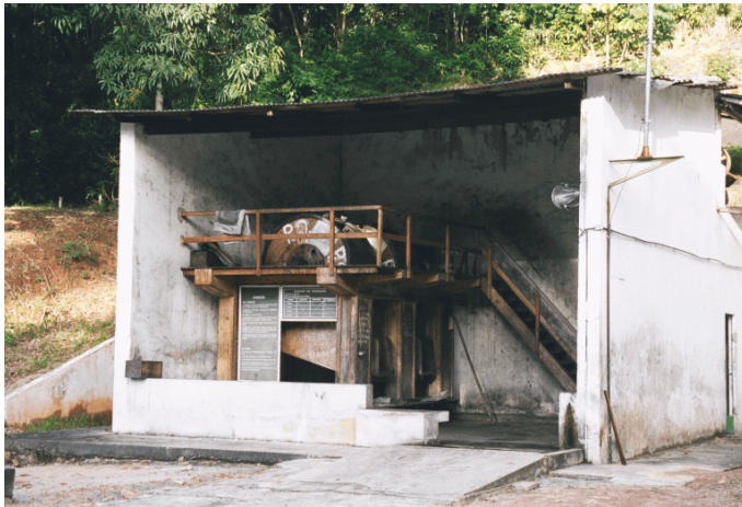
Figure 27. Building housing two polishing barrels.
