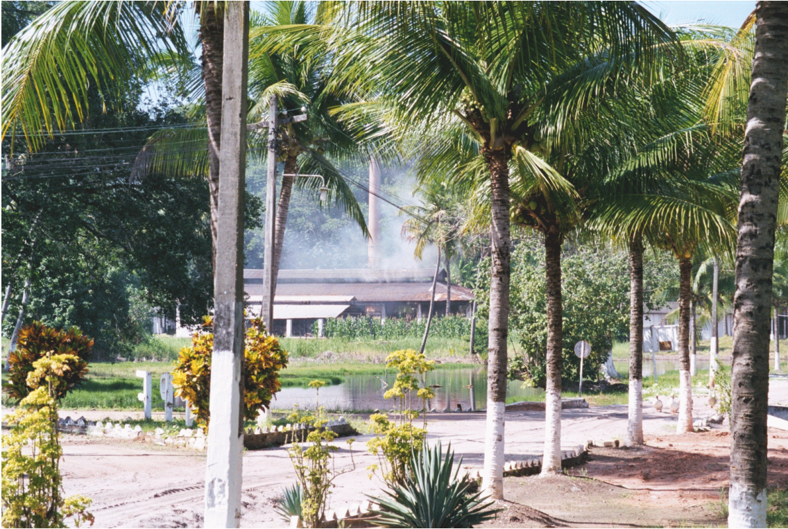
Figure 15. Wood charring building.
