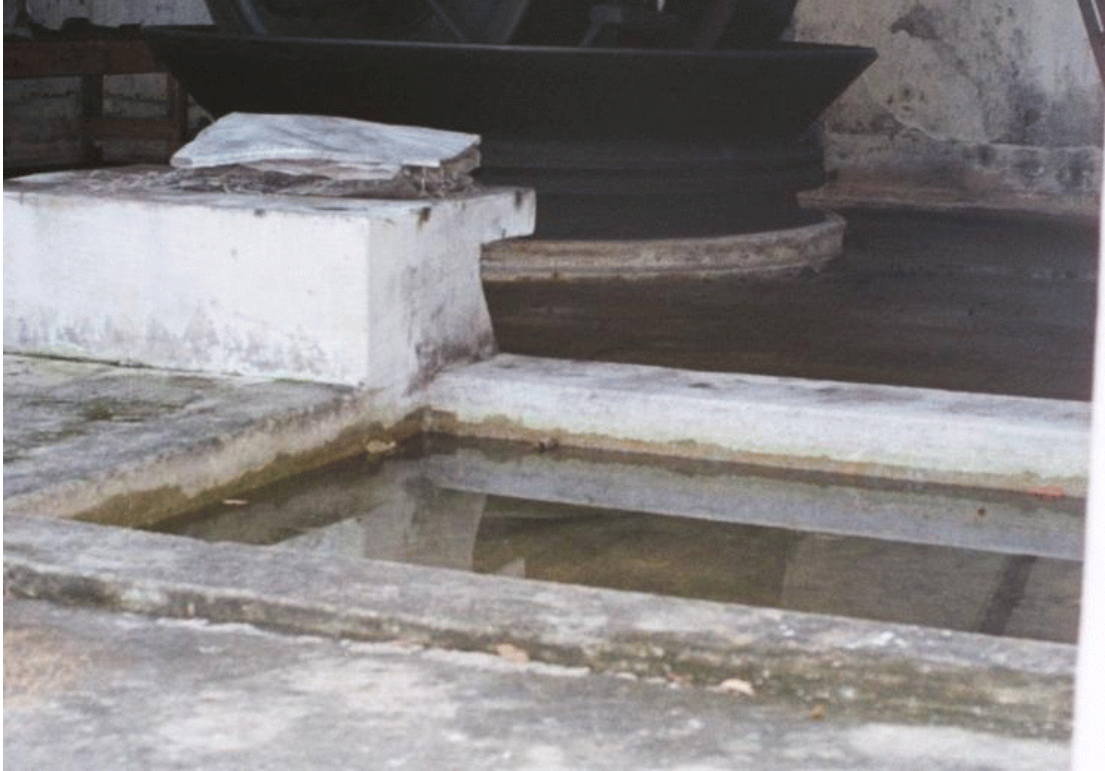
Figure 19. Water pool at the entrance to a wheel mill building.
