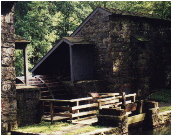
Figure 28. Water wheel and water flow gates.
