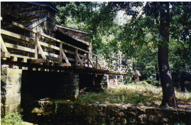
Figure 26. Wheel mill servicing bridge.
