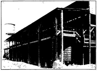
FIGURE 64. Boiling Tubs for Purification of Nitrocellulose.
