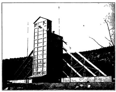
FIGURE 77 Smokeless Powder Blending Tower The powder is blended by being made to flow through troughs and bins Lots as large as 50,000 pounds of rifle powder and 125,000 pounds of cannon powder have been blended in this tower.
